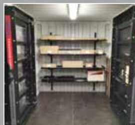
Storage for spare parts
