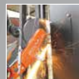
Quick saw & Chain Saw Breaching
